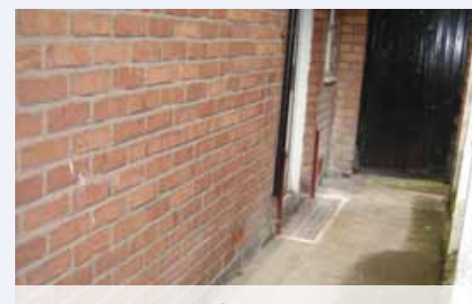
Figure 4 Door guard fixtures and auto-closing airbricks on a house in Dallam
